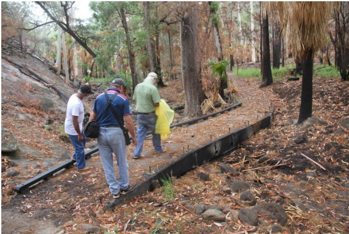
Figure 4: The plastic guardrail on the right that once was in the fire's path burnt and melted.
