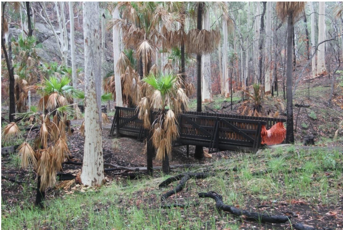
Figure 5: Wooden bridges, although scorched, survived largely intact, unlike plastic infrastructure.
